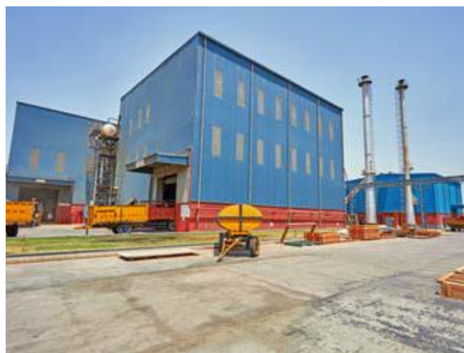
■ Biomass Based Steam power system, Rohad
