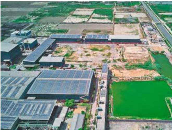
■ Rooftop Solar, Rohad
