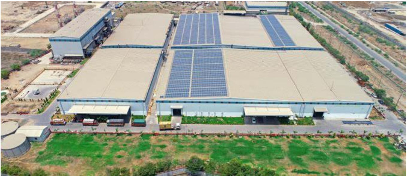
■ Rooftop Solar, Dahej
