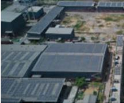
■ Rooftop solar system at Rohad unit
