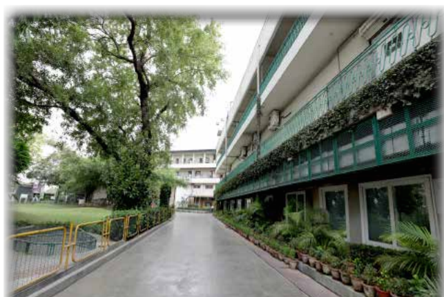
Administrative Block at Factory- MIL Hapur
